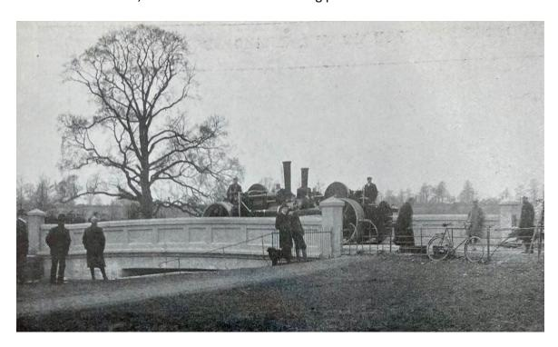
The article mentions that the foundations, abutments, deck, and parapets were all of ferro-concrete, and that the cost compared very favourably with masonry and steel girder decking. And, the ferro-concrete had the additional advantage of not requiring painting or maintenance.
